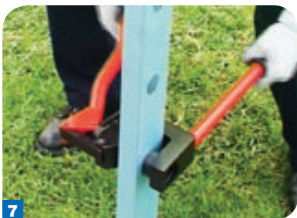
7 A hand punch for light gauge steel is used to create the pilot hole.
