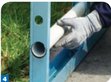
4 The same hydraulic tool is used to make smaller holes for water pipe and electrical cable.
