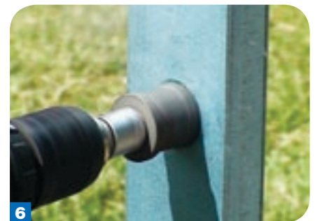
6 A larger pilot hole is required for the bigger handle. In this case, use a water pipe-size punch or cutter.
