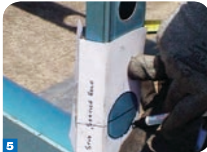
5 When cutting a penetration hole in a boxed stud, use a pre-made template to position a hole at your measured line on either side of the stud. Mark the holes on both sides.
